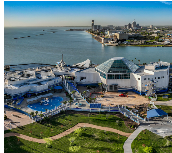
Texas State Aquarium draws over 500,000 annual visitors. Fiber connectivity is key to their outreach strategy.
