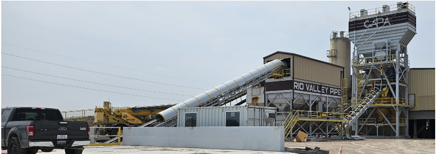
CAPA plants need to be able to run continually, without disruption. Helping them do just that is a Service Level Agreement (SLA) with Spectrum Business guaranteeing 100% uptime.
